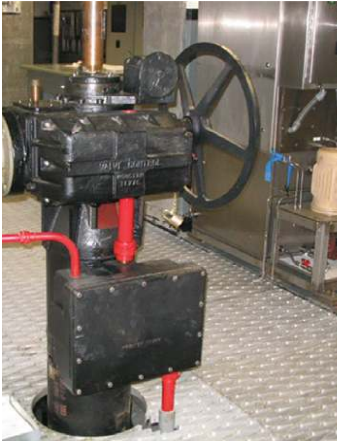
Current M2CP units evolved from proven technology—as shown by this EIM actuator, still operating after more than 50 years at a water distribution and storage system in New York City.
